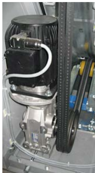
DESI rotor cassette with drive
